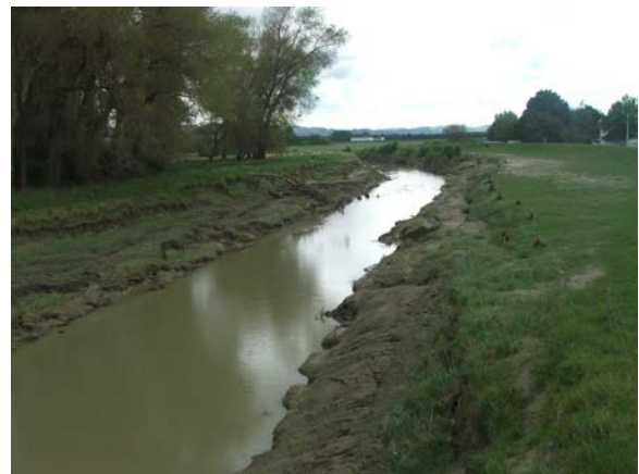
From SH Bridge looking east
